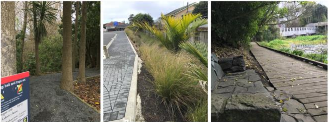
Permeable gravel surface at an entrance to Van Damm's lagoon minimise damage to existing ti kouka (cabbage trees) (left); a swale at the carpark uses native sedges (centre); a broad boardwalk has improved safety and sewer is covered (right).
