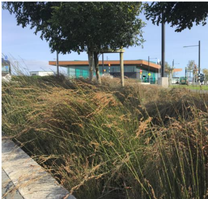
This large raingarden with healthy titoki trees adjacent to the bus station has low maintenance due to dense groundcover and relatively large core relative to edge (left); trees in this small 'island' raingarden in the park and ride have died; surviving oioi groundcover (sedges were inadvertently killed by glyphosate spray) has been over-trimmed, exposing large areas of bare soils (right)
