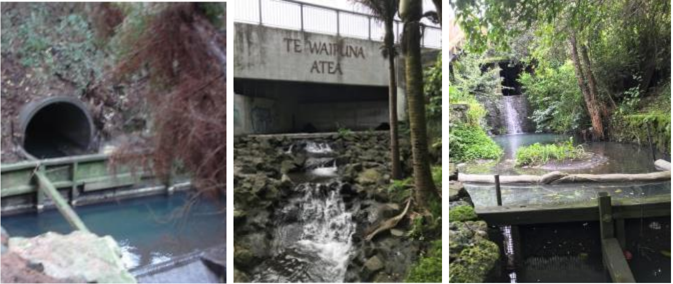
Inlets in 2010, before works (left) and after works in 2018 with naming, waterfall and hidden energy dissipation structure under the bridge (centre). A second inlet has stonewalls flanking a litter screen and oil & grease bund, both of which require regular maintenance to minimize short-circuiting (right)
