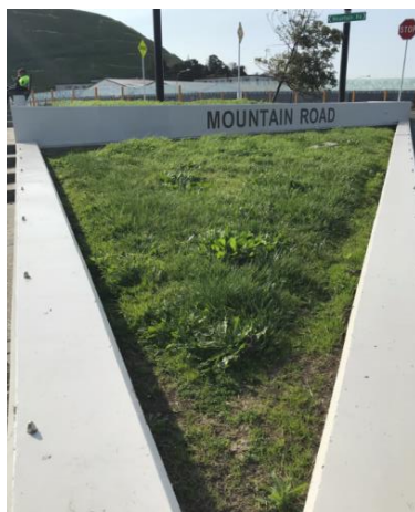
Turf platforms that are expensive to maintain (left); deep raingardens on Potaka Lane have healthy kohekohe trees that need trimming to retain sightlines, the wide inlets are resistant to being blocked by sediment and easy to clean but some are redundant (centre); these grassed areas on Quinlan Street cannot be mown so are maintained with regular herbicide sprays that creates poor aesthetics.
