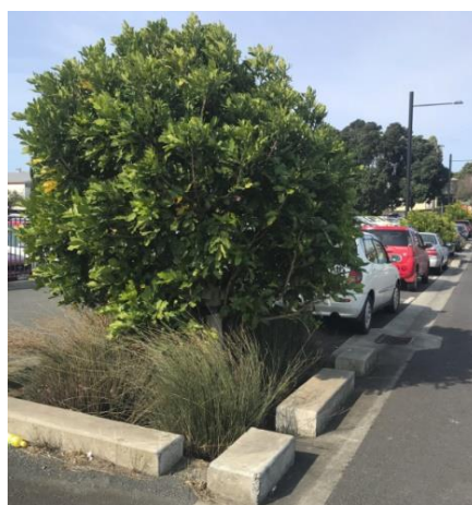
Turf platforms that are expensive to maintain (left); deep raingardens on Potaka Lane have healthy kohekohe trees that need trimming to retain sightlines, the wide inlets are resistant to being blocked by sediment and easy to clean but some are redundant (centre); these grassed areas on Quinlan Street cannot be mown so are maintained with regular herbicide sprays that creates poor aesthetics.
