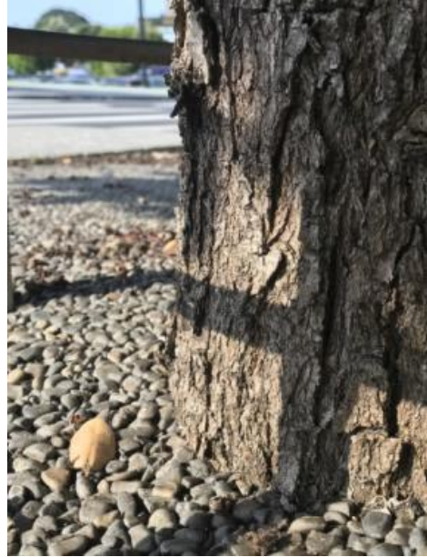
Tree pits with poured-resin permeable paving could have been used to treat road runoff (left); the resin needs regular removal to avoid ringbarking the growing tree (right)
