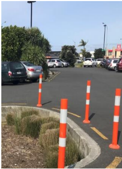
This large raingarden with healthy titoki trees adjacent to the bus station has low maintenance due to dense groundcover and relatively large core relative to edge (left); trees in this small 'island' raingarden in the park and ride have died; surviving oioi groundcover (sedges were inadvertently killed by glyphosate spray) has been over-trimmed, exposing large areas of bare soils (right)
