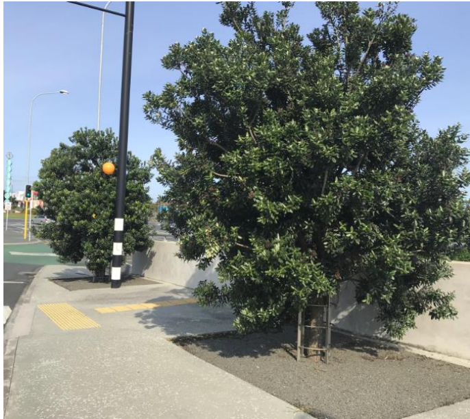
Tree pits with poured-resin permeable paving could have been used to treat road runoff (left); the resin needs regular removal to avoid ringbarking the growing tree (right)
