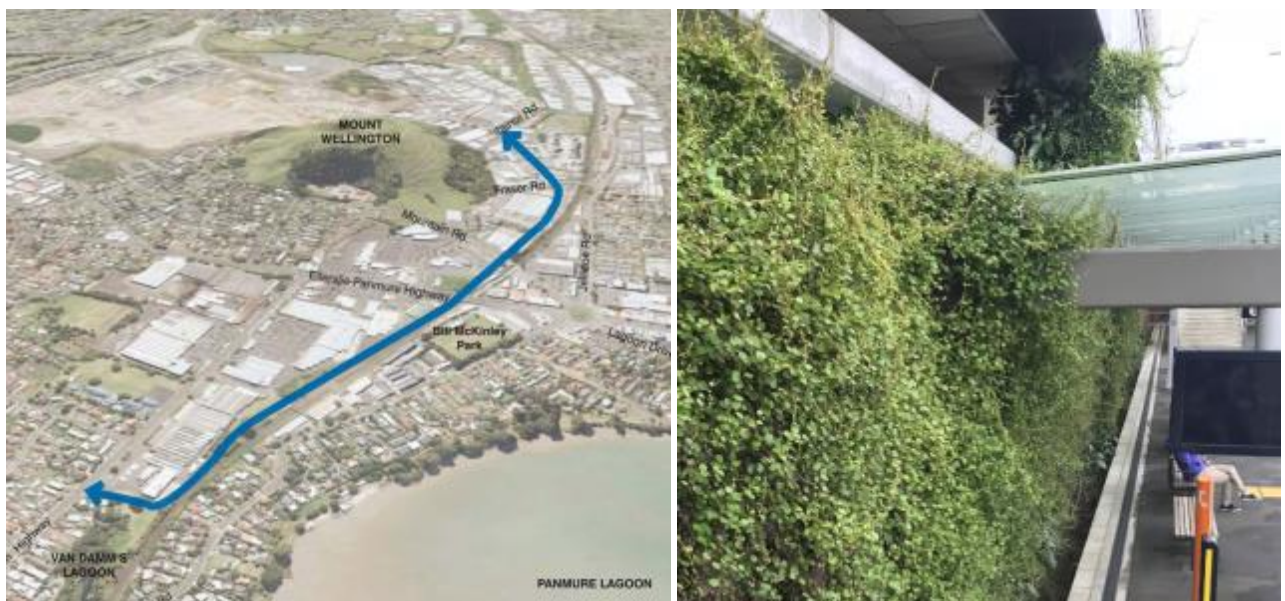
AMETI Stage 1 (design 2011) and green screen in stormwater planter boxes at the Panmure railway station (2018)
