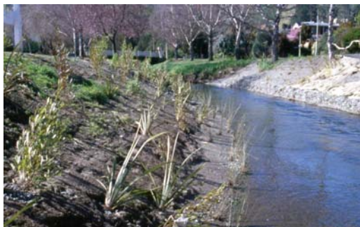
■ An example of river bank rehabilitation at Christchurch's Heathcote River. The eroded bank was recontoured and replanted with rushes, sedges, New Zealand flax, cabbage trees, and other suitable native plants.
