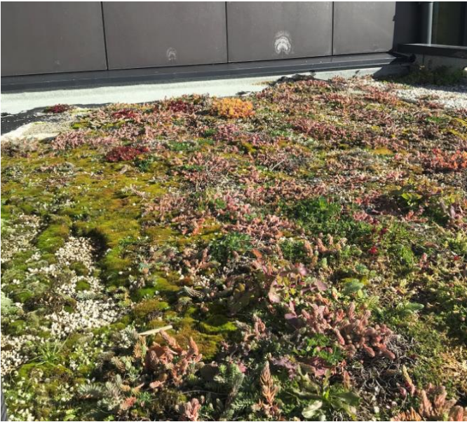
Left: The pale strip at the base of the wall is the waterproof membrane that has been exposed by wind-scour of the thin media. Salting of the roof may also have had an effect. Right: Bright-green mosses have established in some places and are very tactile.
