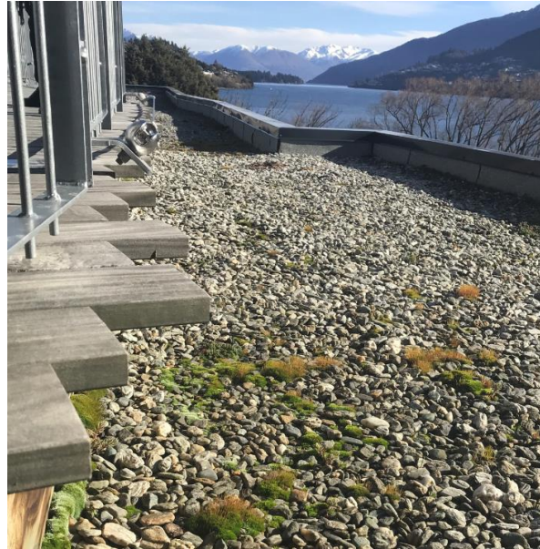
Left: The pale strip at the base of the wall is the waterproof membrane that has been exposed by wind-scour of the thin media. Salting of the roof may also have had an effect. Right: Bright-green mosses have established in some places and are very tactile.
