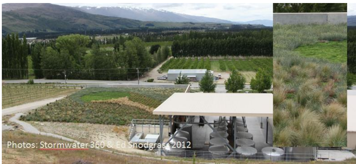
Mt Difficulty roof after about 12 months when thyme was still a dominant feature
