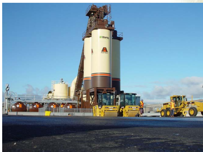
Works Infrastructure’s asphalt production plant at Mt Wellington.
