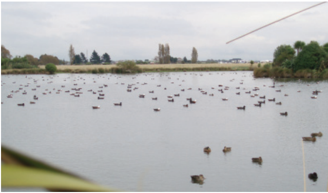
FIGURE 4 Wigram Retention Basin, Christchurch, at commencement of duck-shooting season – demonstrating the multi-purposes of flood attenuation and water filtration (raupō beds) from the Sockburn industrial estate with wildlife refuges (paradise shelducks and grey teal).
