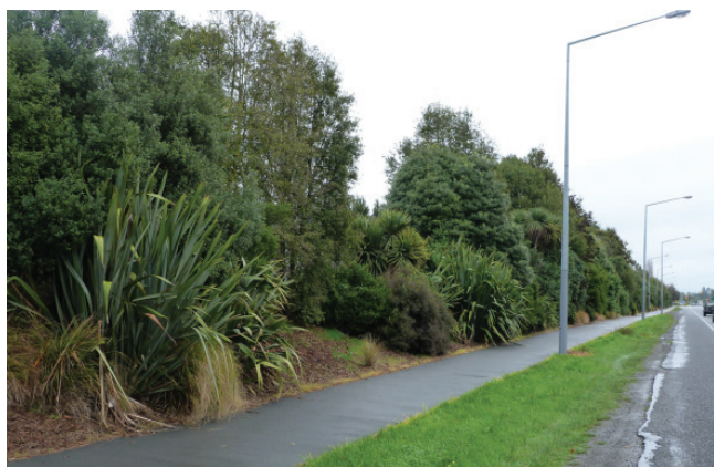
FIGURE 6 Noise and air pollution buffer separating residential property and Queen Elizabeth II Expressway, Northwest Christchurch with high biodiversity corridor values. This is a combination of a 3m high earth embankment (main noise barrier) planted with forest species to muffle the noise: Plagianthus (lowland ribbonwood/mānatu), Pittosporum (kōhūhū and lemonwood/tarata), Coprosma (karamū and mikimiki), Griselinia (broadleaf/kāpuka), Cordyline (cabbage tree/tī kōuka), Dodonaea (akeake), Sophora (kōwhai), Phormium (NZ flax/harakeke), Pseudopanax (five-finger/whauwhaupaku), Olearias and Hebe (koromiko) and Anemanthele (wind grass).
