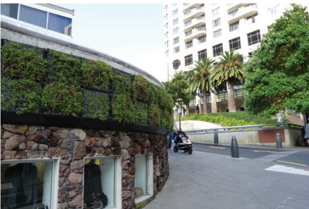
FIGURE 8 (Top) Green roof, (middle) porous paving (Ellerslie International Flower Show Exhibit), and (bottom) living wall (Auckland) – aesthetically calming water attenuation devices for urban environments.
