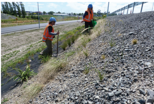
FIGURE 9 Establishing locally rare dryland species (e.g. Dichelachne , Lachnagrostis , Geranium , Leptinella , Muehlenbeckia ) in a specially prepared stressed niche (very-free-draining, north-facing substrate) on the Christchurch Southern Motorway extension.
