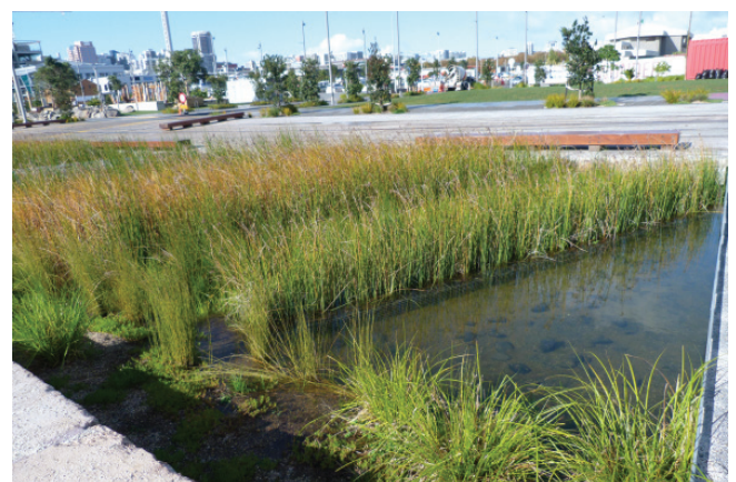
FIGURE 5 The Wynyard Quarter, Auckland City waterfront, demonstrating good urban design with rain gardens and wetland treatment for recreation, biodiversity and stormwater purification before water enters the harbour.
