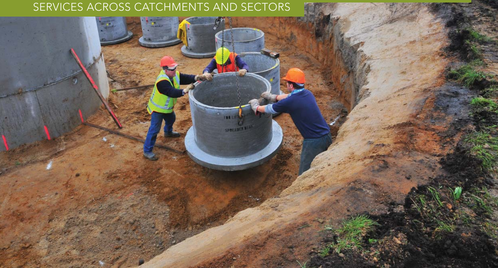
Installing lysimeter casings at the large scale array near Lake Taupo.
