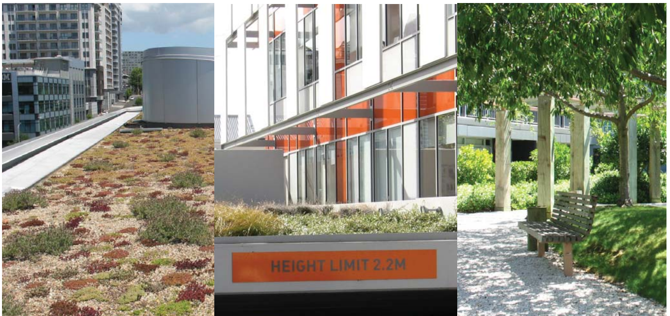
New Zealand green roofs (from left to right) increasing in cost, weight, soil depth, plant height, water requirement and maintenance. (Left to Right) A lightweight green roof of 100-mm-deep 'soil' with succulents (not irrigated) to irrigated 300-mm-deep 'soil' (garden) to 500-mm-deep 'soil' (where small trees are placed).
