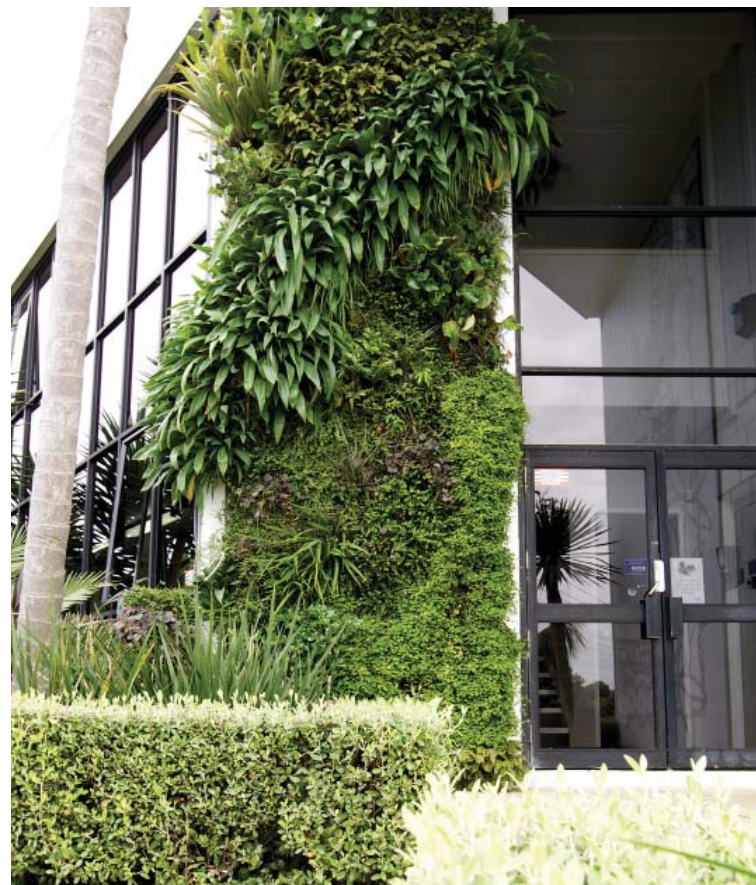
Exterior native living-wall, now relatively low maintenance except for irrigation and occasional stripping.
