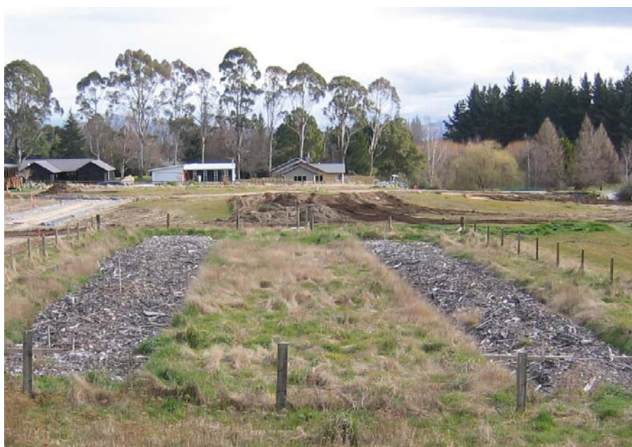
■ Twin denitrification beds near new suburban development at Kinloch. This photo was taken in 2003 when the beds were first installed.
