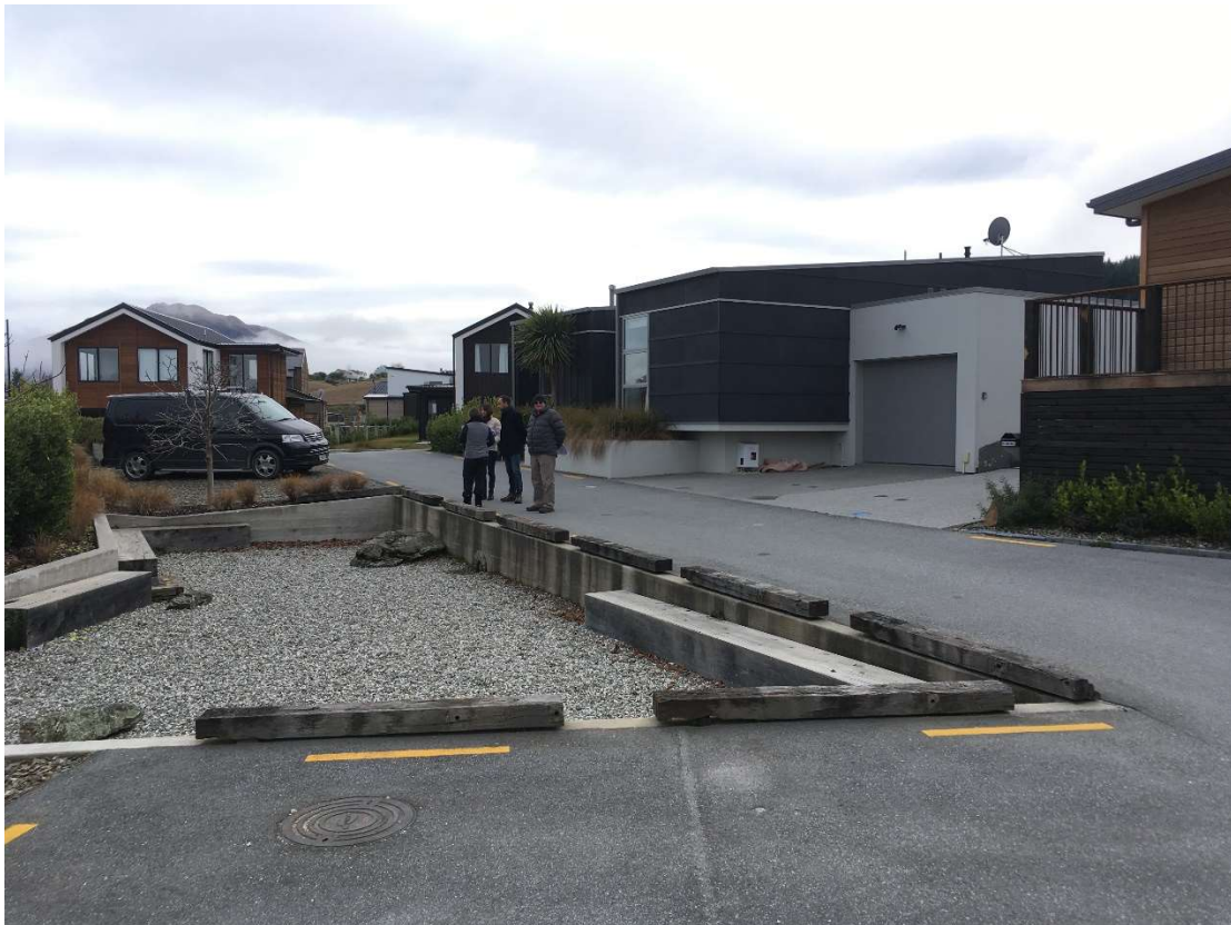
Figure 4-1 – Photos of the KiriMoko Park development showing road and swale design (upper) and stormwater detention area (lower).
