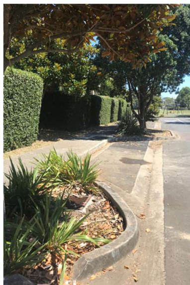
Figure 4-7 – Photos/plan of the Talbot Park re-development showing the area before redevelopment and as redesigned (source: Boffa Miskell, 2005) (upper) and road side rain gardens (lower).
