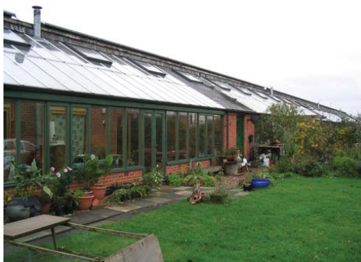
■ An example of sustainable housing: The Hockerton Housing project designed by Brenda and Robert Vale and completed in 1998. Among its energy-saving features are solar panels, triple glazing, and food-growing areas.
