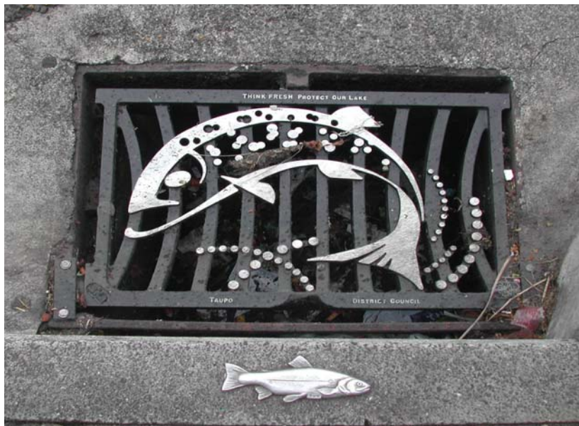
More fun for fish: this decorative drain in Taupo not only looks good, it contains mesh to prevent rubbish from entering waterways.
