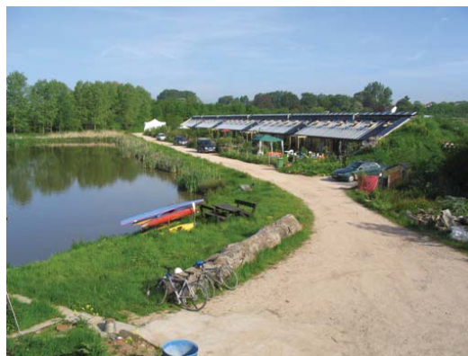
■ An example of sustainable housing: The Hockerton Housing project designed by Brenda and Robert Vale and completed in 1998. Among its energy-saving features are solar panels, triple glazing, and food-growing areas.
