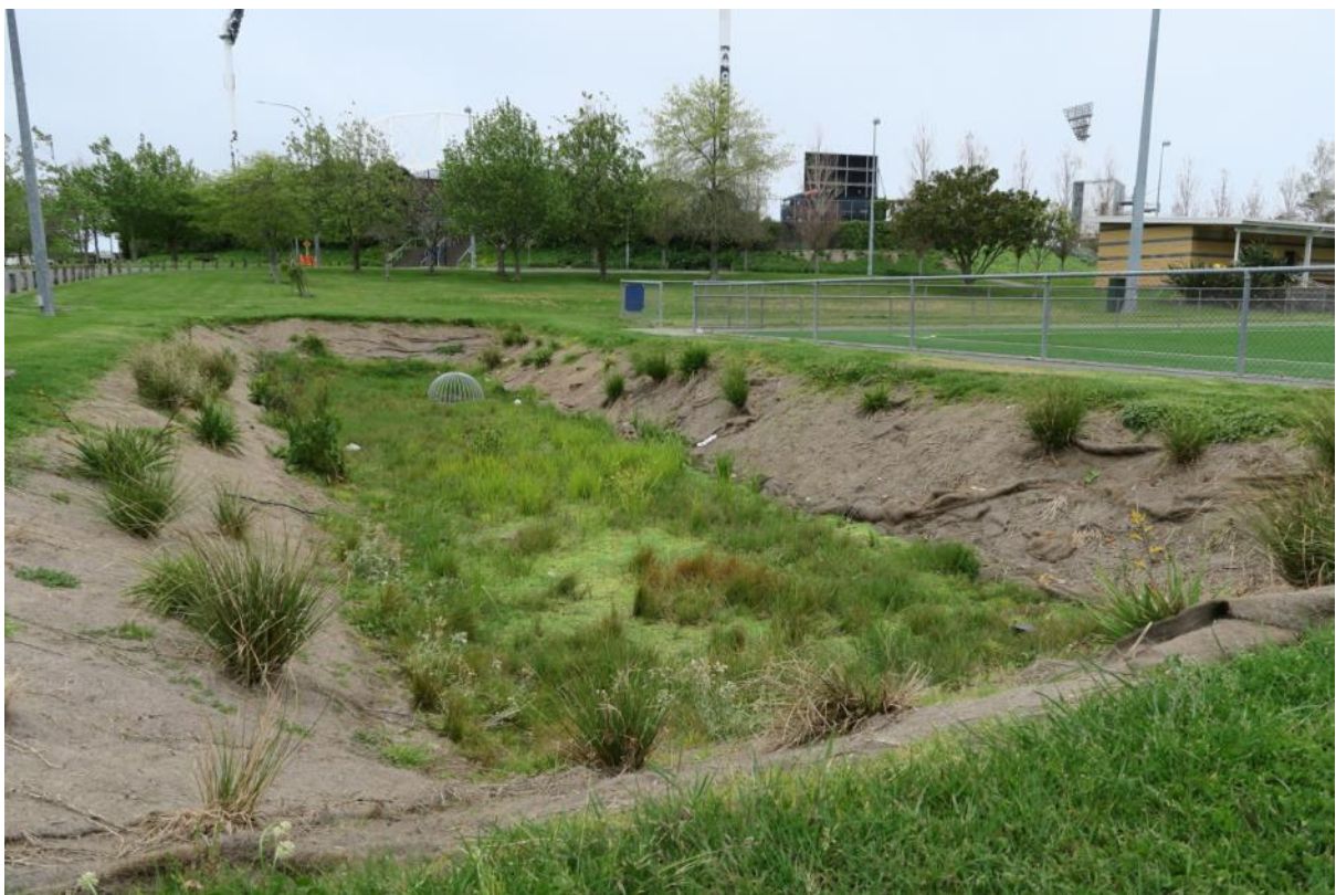
Ugly detention basin / raingarden receiving runoff from artificial turf: High maintenance, narrow benefits
