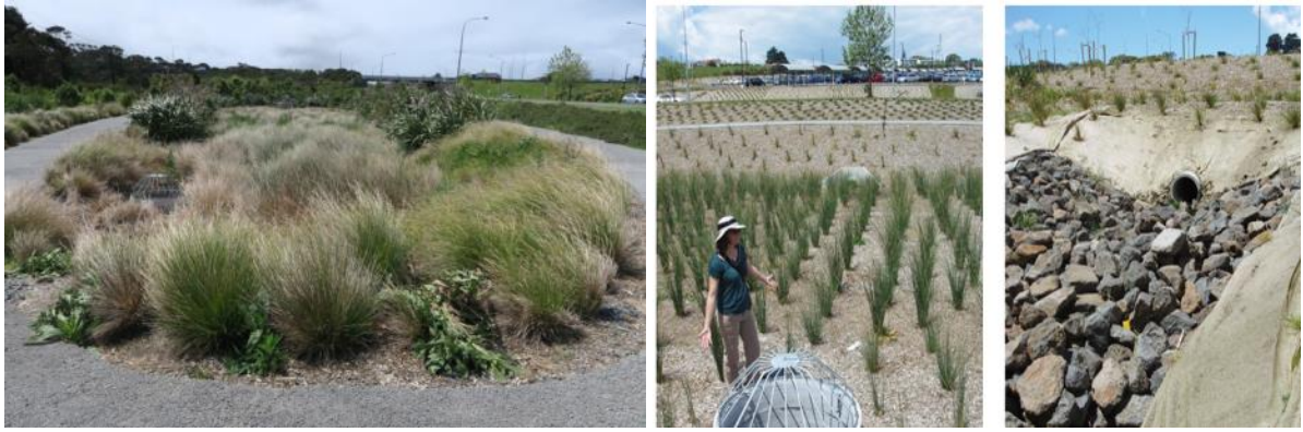
Albany park and ride station large raingarden (part of treatment train). Right photos are from 2012 and show overflow and rock-lined outlet structures
