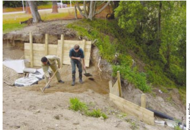
Surya Pandey and Matthew Taylor of Landcare Research, preparing the ground for monitoring equipment to be installed next to an experimental treatment wall.
