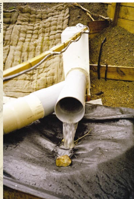
Road run-off discharging into the treatment wall structure.
