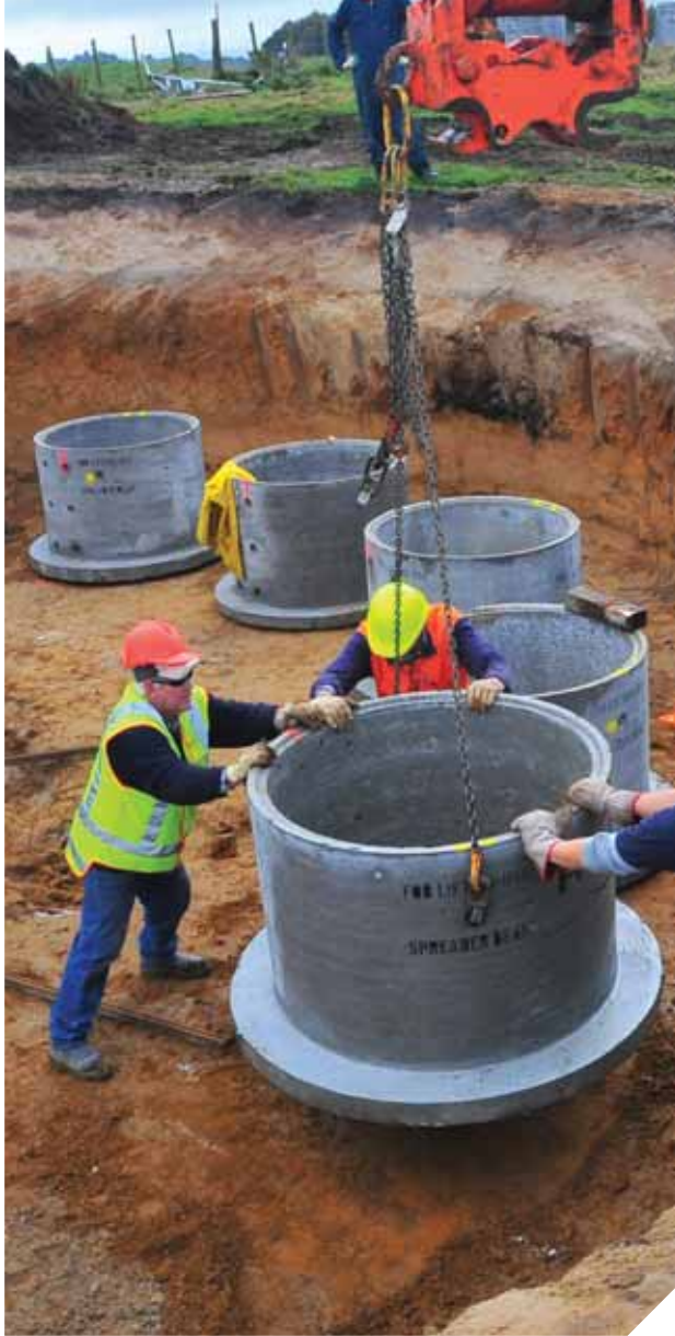
Installing lysimeter casings at the large-scale array near Lake Taupo
