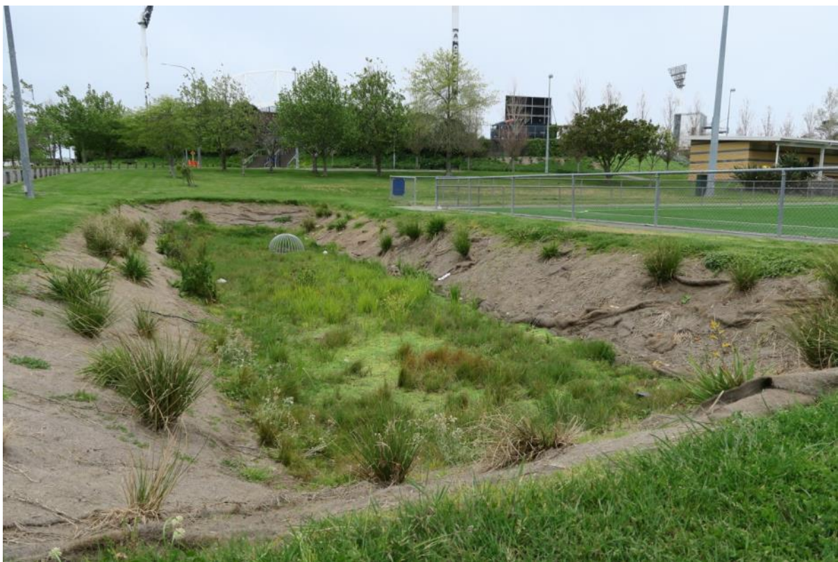
Ugly detention basin / raingarden receiving runoff from artificial turf: High maintenance, narrow benefits
