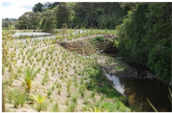
Lucas Creek reshaping of flood zone and riparian area to reduce erosion/bank instability by increasing floodplain width, adding habitat features (right photo is 2012)
